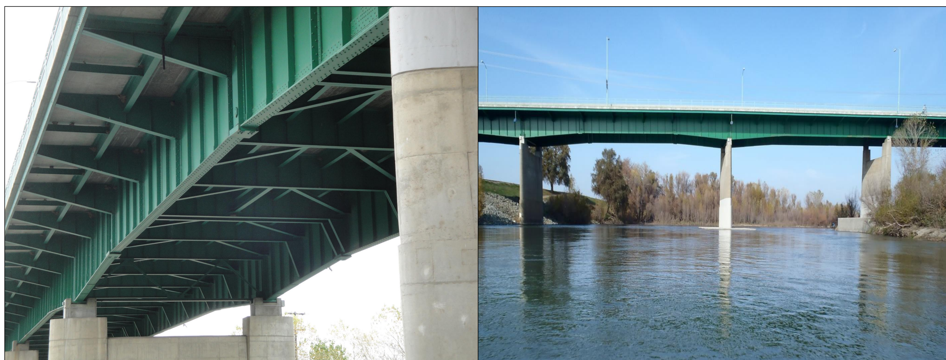
Figure 1. Side views of the main spans from the Feather River Bridge
