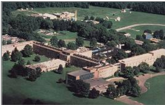
Sarnoff headquarters, Princeton, NJ
